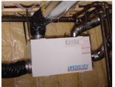
Although this option costs \$2000 to \$2500 installed, it will fix your wet window problem once and for all. It will also retain most of the heat that you'd normally lose through open windows and out of exhaust fans. In fact, HRV's are
