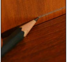
Most laminate installations involve areas covered by the arc of a swinging door, and even though laminates are relatively thin, you'll probably still need to trim the bottom of your doors to accommodate the raised floor.
