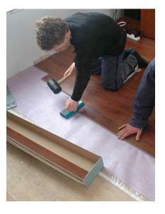
using gentle blows with a rubber mallet driving a tapping block (see below, left). Keep the force of each blow light, and stop pounding as soon as the end joints are tight. Overdriving boards can cause joints to open up in other parts of the floor.
