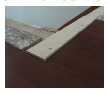
A flush, smooth joint is my favorite way to make the transition between a laminate floor and the top tread of a staircase. To make this happen, install a temporary plywood strip where you want the laminate to end, then butt the laminate up against this strip as you secure each piece. Make smooth end cuts on the laminate using a chopsaw, using a special carbide blade, then sand a slight bevel along the top edge of
